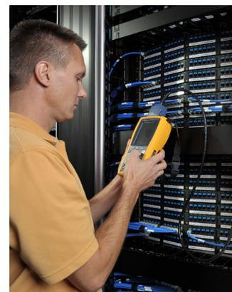
Terrance Electric used Fluke Networks’ DTX CableAnalyzer to certify the new installation to 10GBASE-T. Multiple two-man teams were used to test and document over 40,000 links.
